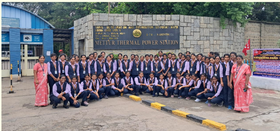
Mettur Thermal Power Plant visited by Third Year Students and Faculty Members on 18-09-2025
